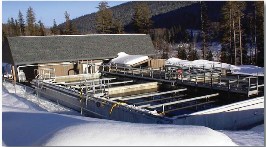
Sun Peaks wastewater treatment plant – Phase 1
