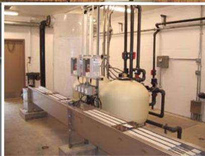
*Mechanical room - sand filters and UV disinfection.*
