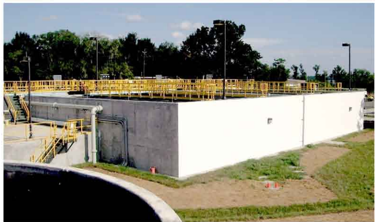
City of Lake Alfred, FL USBF™ WWTP - IMGD (4,000m 3 /d)
