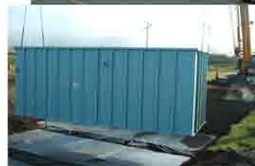
80,000GPD (300m 3 /d) packaged municipal USBF™ WWTP installation in Northern BC, Canada.
