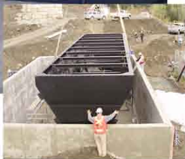
375,000GPD (1,400m 3 /d) ski resort USBF™ WWTP - highly fluctuating flows. Modular expansion (right).
