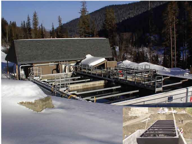
375,000GPD (1,400m 3 /d) ski resort USBF™ WWTP - highly fluctuating flows. Modular expansion (right).
