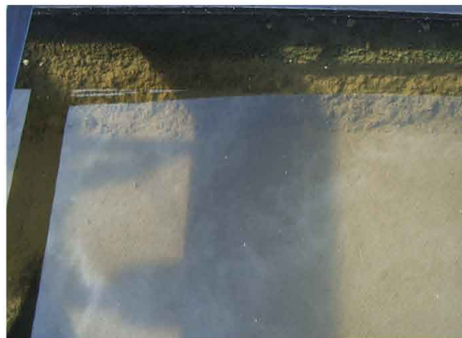
High quality USBF™ effluent at the surface, filtered up through the sludge blanket (intentionally raised).
