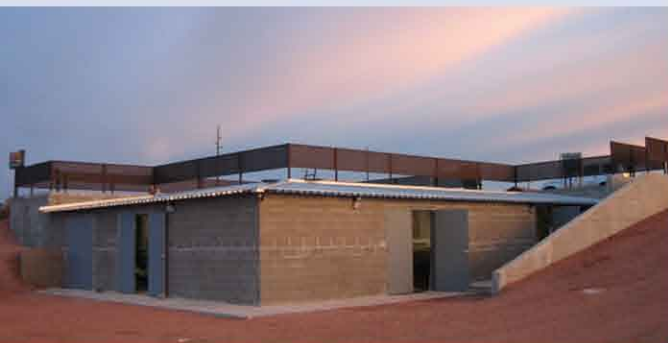
80,000GPD (300m 3 /d) USBF™ WWTP. Water reused for irrigation and fire suppression at nearby hotel/casino.
