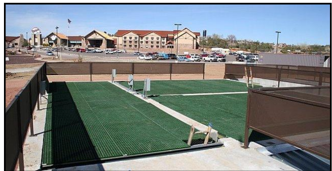
Notice the close proximity of the WWTP to the casino/hotel, attesting to the non-odorous nature of the USBF process
